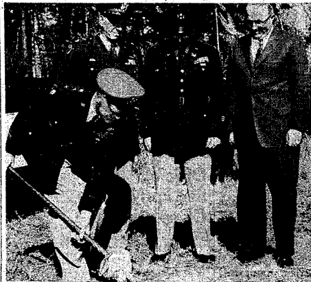
FIRST SHOVELFUL . . . Major General Herbert B. Powell, foreground, Infantry Center commander, initiated the construction of $14 million worth of Capehart housing on post Feb. 1 by turning the first shovel of earth with a gold-plated shovel on are, left to right, Major Gen. George E. Lynch, 3rd Inf. Div. commander, Col. R. C. Bahr, district engineer of the U. S. Army Engineer District, Savannah, Ga., and C. Edwin Gates, president of Williams Construction Company, Columbus, Ga.
