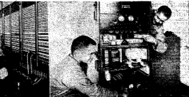
Left to right are: SFC Dennis Anderson, Pfc. Donald Craig and Pfc. Robert Gilchrist. At right: Pfc. James W. Coody and Sgt. Joseph F. Hanzel. check power supply to the new-installed 220-
