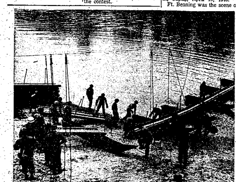
RIVER CROSSING... Members of the 586th Engineer Co. are shown supporting a river crossing problem. This type of bridge is the aluminum foot bridge.
